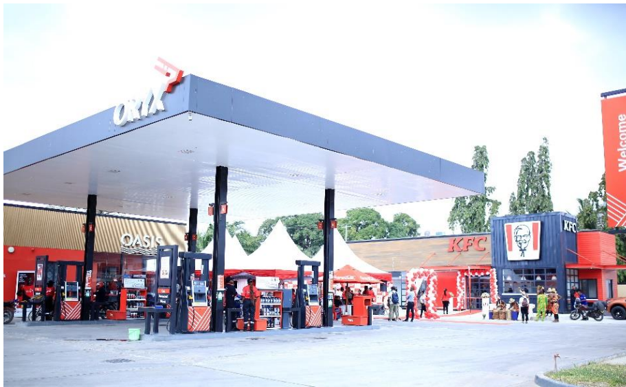
ORYX Morocco service station, Dar-es-Salaam with KFC Drive-Thru and BAO Café
